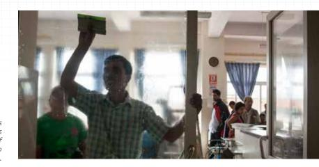
Ensuring hospitals remain operational after an earthquake is critical for post disaster response and recovery. FLAGSHIP 1 is supporting efforts to strengthen the operational capacity of hospitals. In this photo, a worker is adding glass protection to prevent shattered glass.
